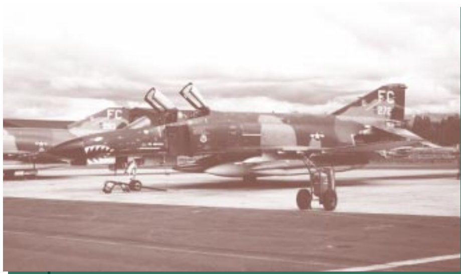
The F-4E "Phantom II" was deployed to Alaska in 1970. The F-4E had a maximum speed exceeding mach 2, a range of 2,300 miles, and a combat ceiling of 71,000 feet. This high-powered aircraft was responsible for increasing the number of intercepts of Soviet aircraft despite a reduction in interceptor squadrons.
